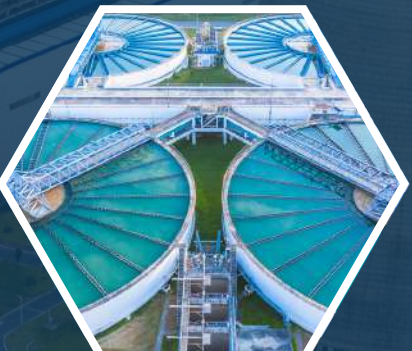
Water & Wastewater Treatment
