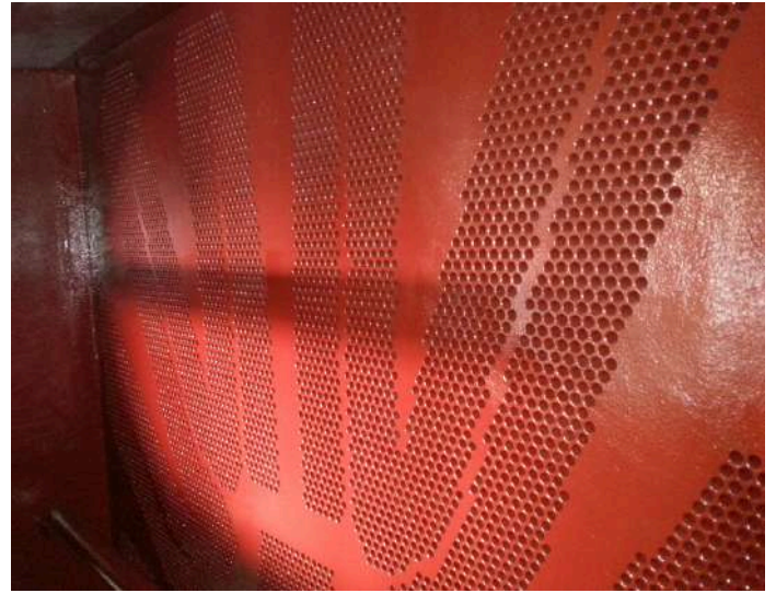
Heat-Exchanger Tube Sheet protected using plastocor® Cladding system.
