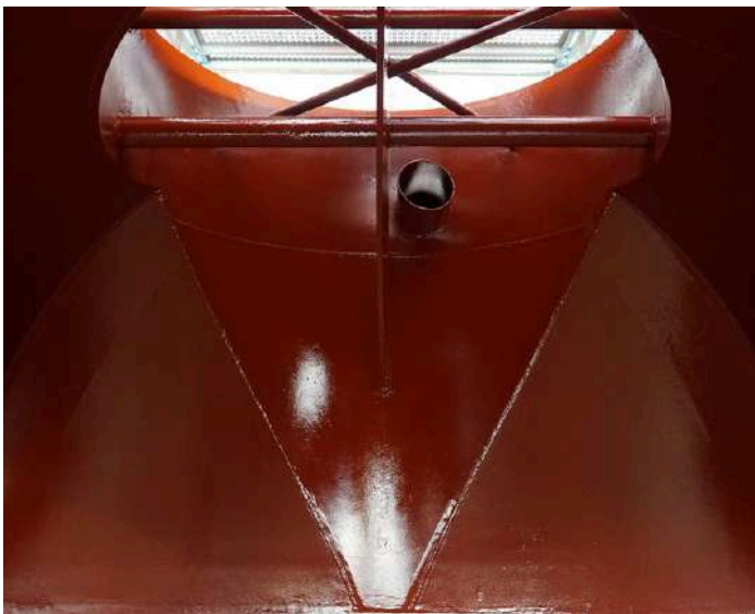
Heat-Exchanger Water Box coated using plastocor® High-Performance Coating System
